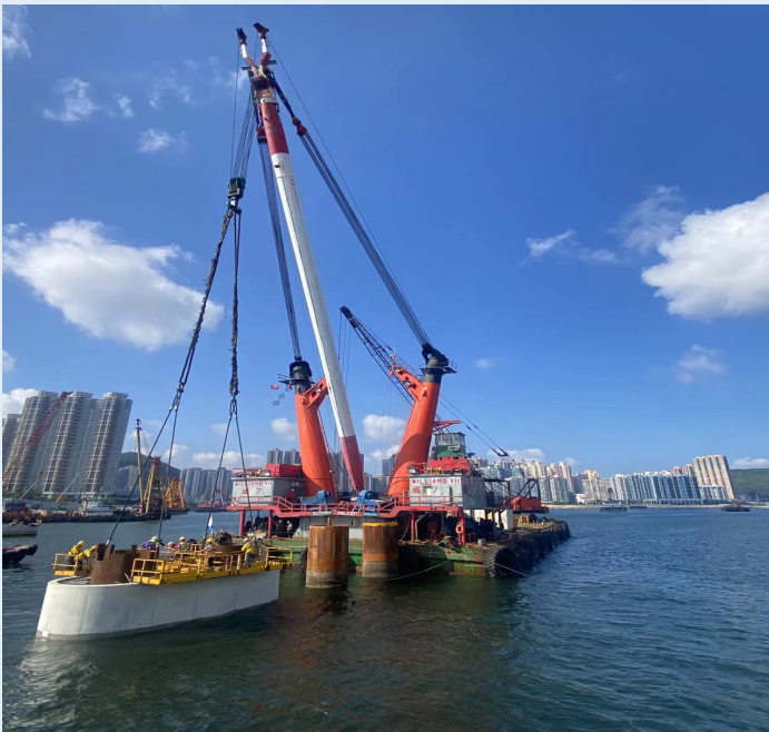
香港将军澳大桥吊装水下桥墩 Lifting Installation of Underwater Piers of Tseung Kwan O Bridge, HK
