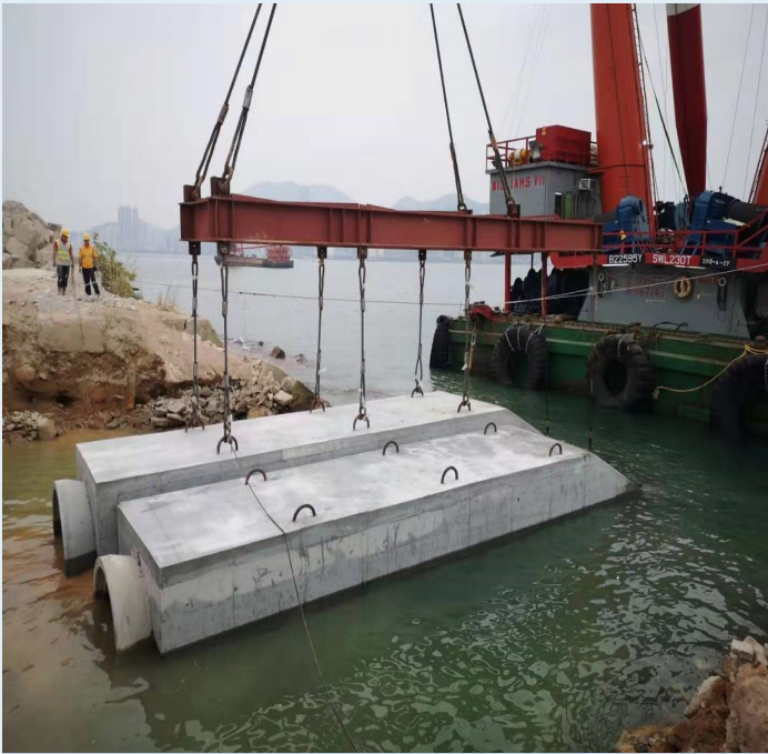
香港启德预制件安装 (2019) Lifting Installation of Precast Blocks at Kai Tak, HK
