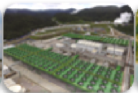
Sarulla Geothermal Plant (110MW) Indonesia (2016 – 2017)
