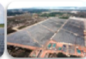
LIG Quang Tri plant, 50MW Vietnam (2019)
