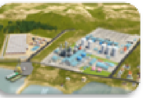
Melaka CCGT Plant (2,242 MW) Indonesia (2018-2019)
