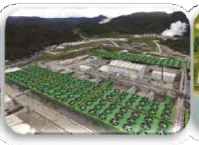
Sarulla Geothermal Plant (110MW) Indonesia (2016 – 2017)
