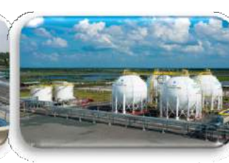
Ca Mau gas processing plant Ca Mau, Vietnam
