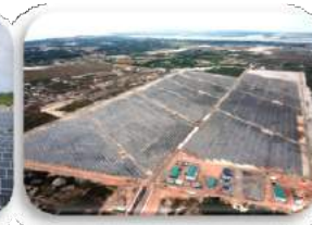
LIG Quang Tri plant, 50MW Vietnam (2019)
