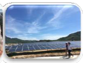
Cam Lam plant, 50MW Vietnam (2019)
