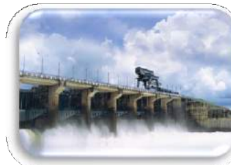
Tri An plant, 400MW Dong Nai, Vietnam (2003)
