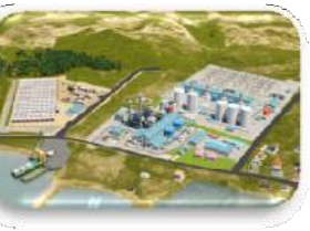
Melaka CCGT Plant (2,242 MW) Indonesia (2018-2019)
