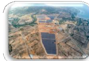
Gelex plant, 42MW Vietnam (2018)
