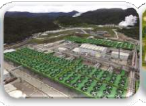
Sarulla Geothermal Plant (110MW) Indonesia (2016 – 2017)
