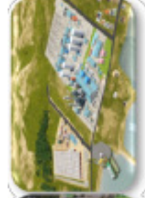
Mela to CCGT Plant (2,242 MW) Indonesia (2018-2019)
