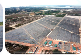
LIG Quang Tri plant, 50MW Vietnam (2019)
