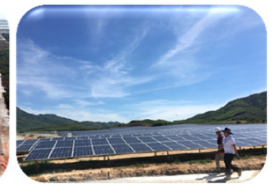
Cam Lam plant, 50MW Vietnam (2019)
