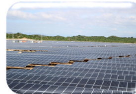
Ninh Phuoc plant, 50MW Vietnam (2019)
