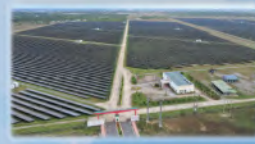
LIG Quang Tri Solar Power Plant (49.5MWp)
