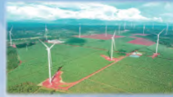
Ia Pet - Dak Doa 1 & 2 Wind Power Plant (200MW)
