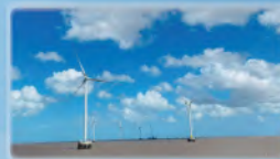
Tan Thuan Wind Power Plant (75MW)
