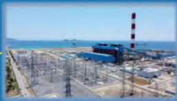
Van Phong 1 Thermal Power Plant and 110kV & 500kV Power Plant Substations (1,320MW)
