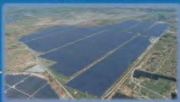
BIM2 Solar Power Plant and Quan The Switching Station (325MWp)
