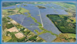
Hoa Hoi Solar Power Plant (257MWp)
