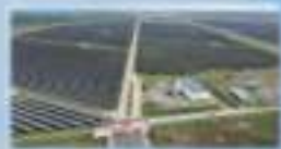
LiG Quang Tri Solar Power Plant (49.5MWp)
