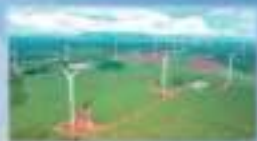
Ia Pét - Dak Doo 1 & 2 Wind Power Plant (200MW)
