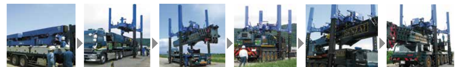
200t all-terrain crane assembly with lifter
