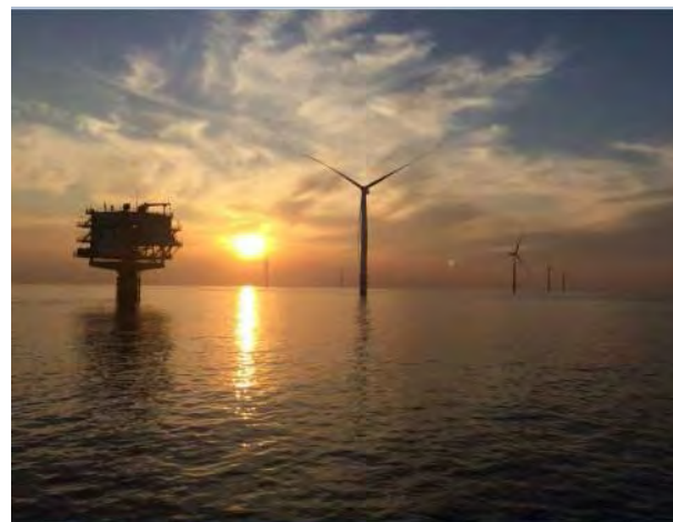
Asia's first 110kV offshore booster station - Rudong 150MW offshore wind project
