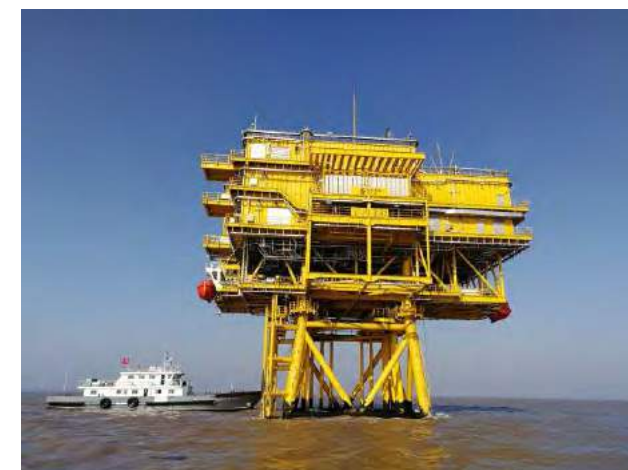
Binhai North H2#400MW Offshore Wind
